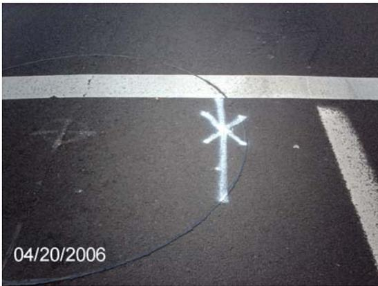
Figure 3. Temporary detection mark.
