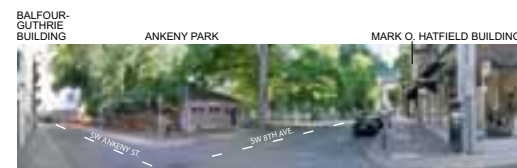
4A VIEW INTO ANKENY PARK FROM STREET CORNER
