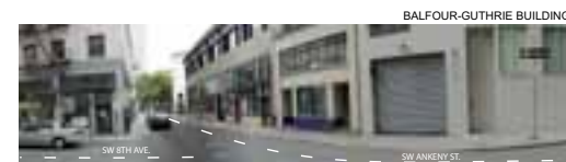
4B VIEW FROM ANKENY PARK AT INTERSECTION
