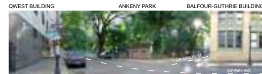
1A VIEW INTO ANKENY PARK FROM STREET CORNER
