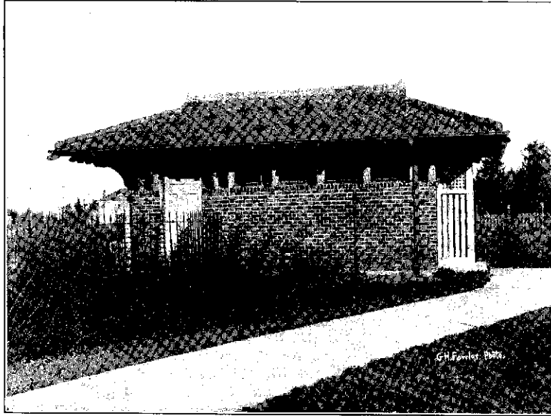
Comfort Station in Peninsula Park
