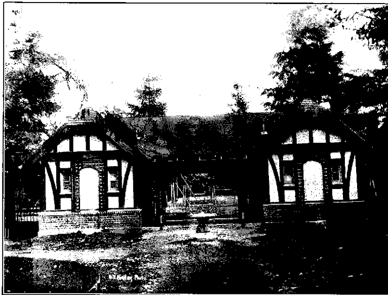
Comfort Station at Columbia Park
