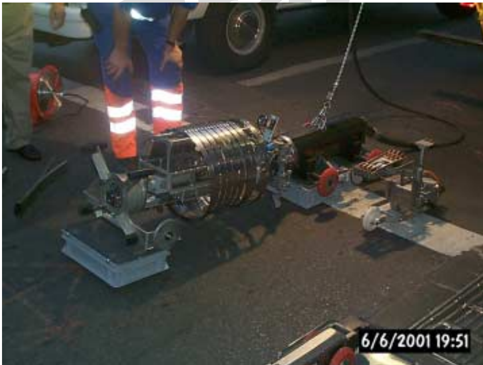
Figure 3. The robot's conduit hanger magazine is loaded with steel bands
