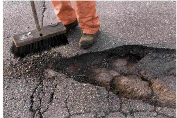
**Pothole on NE Grand Ave, January 2009:** A pothole is a bowl-shaped hole caused by localized disintegration of the pavement surface. Potholes are a structural form of deterioration.
