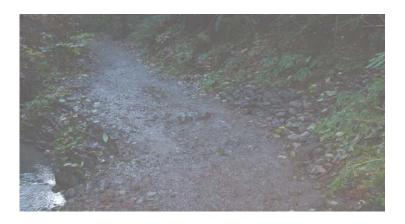
Completed: Install 10ft culvert and dig an inside ditch.
