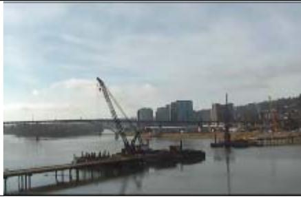
[Base Being Laid For New Willamette River Bridge.](#) "Looking at the site you can see cranes and a lot of barges, but there isn't much bridge. That's because so far, crews are drilling shafts, 140 feet down into the riverbed." *OPB.org, Feb. 23*
